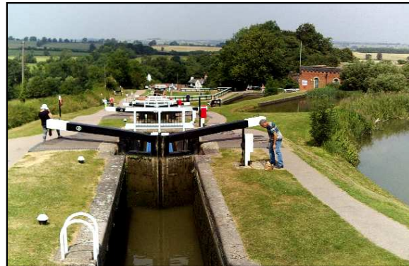
The Foxton lock flight - one of the heritage jewels of the waterways - which needs traditional skills to keep operating.
